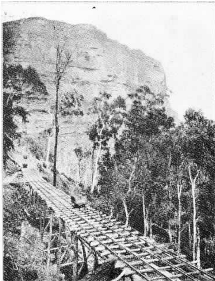
Cable Tramway from Tunnel under Orphan Rock Point and Dog Fi Rock to Narrow Neck Tunnel, about 1894.
