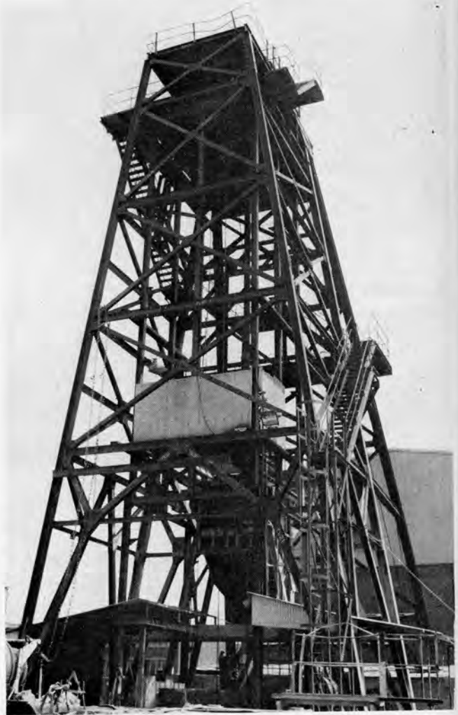
Fig. 1—No. 2 shaft permanent and sinking headgears
