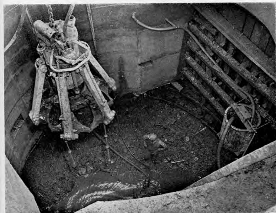
Fig. 2—Looking into shaftcollar— cactus grab on left
