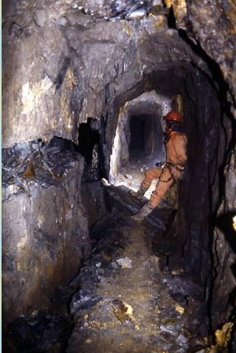
A highly stressed tunnel exhibiting large cracks and fractures in the walls and floor was aptly named "Earthquake Passage." T.L.E. Plan No5.
