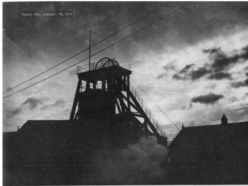
2 Symbol of Coal-Mining: The Shaft with its Great Wheels Wherever coal is mined you see them. Over these wheels passes the cable carrying the cage—in which the miners descend hundreds of feet below the surface to dig out the debris of ancient forests.
