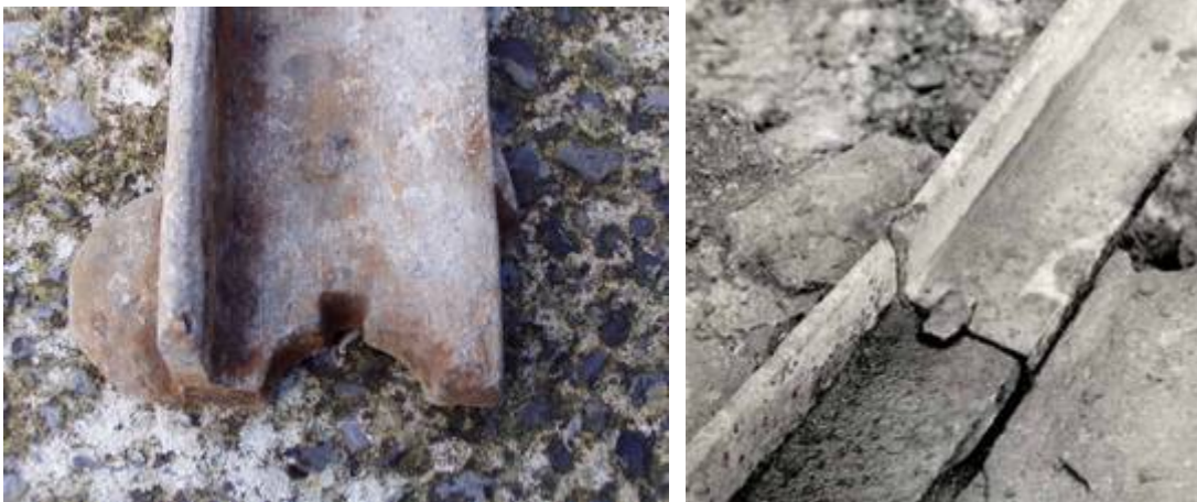
Found at the Grove Colliery the Plateway on the left was fixed to the sleeper by a single pin driven into the slot when they were placed end to end, as shown in the right hand picture.
