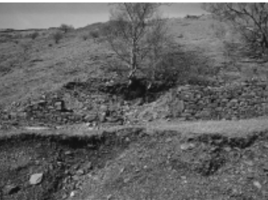
Gilbert's level guardhouse survives to less than half its original wall height. The adit itself is blocked, but is marked by the birch in the centre of the photograph.
